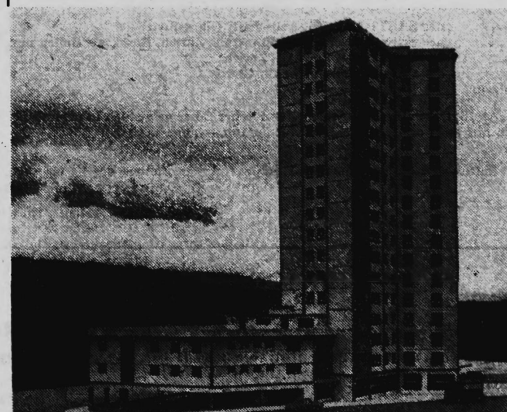
Building Les Charmettes in Frelburg, 17 Stockwerke
