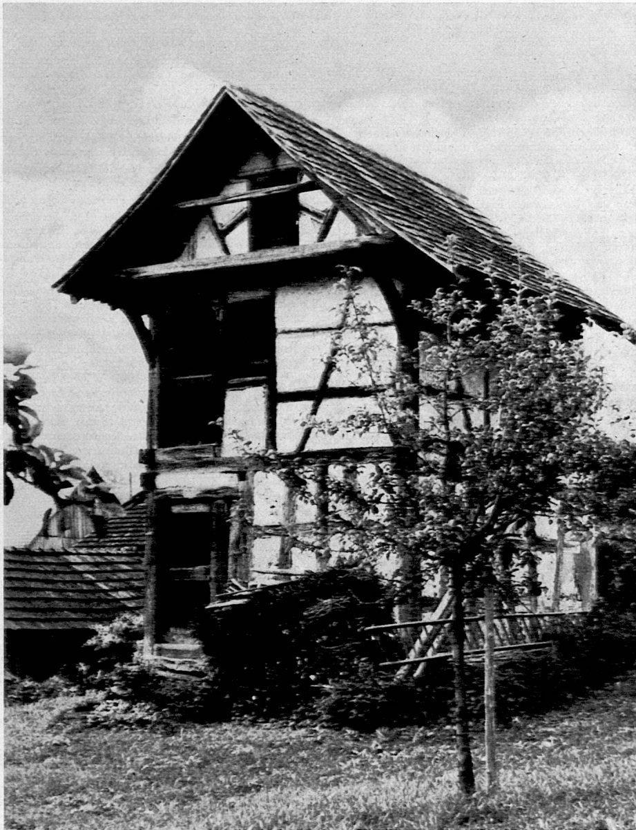
Alter Speicher in Neerach ZH
