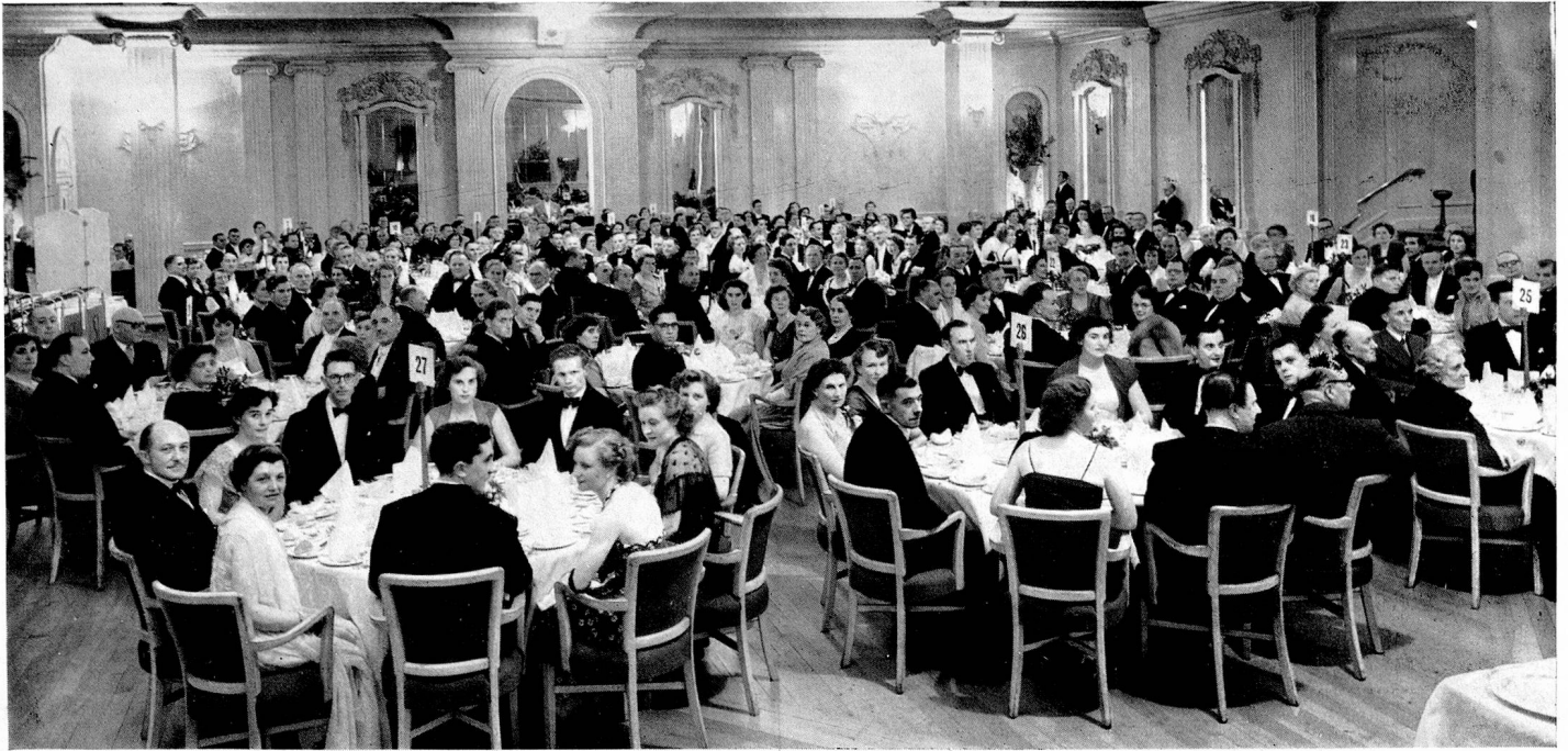
GENERAL VIEW OF THE BALL ROOM.
