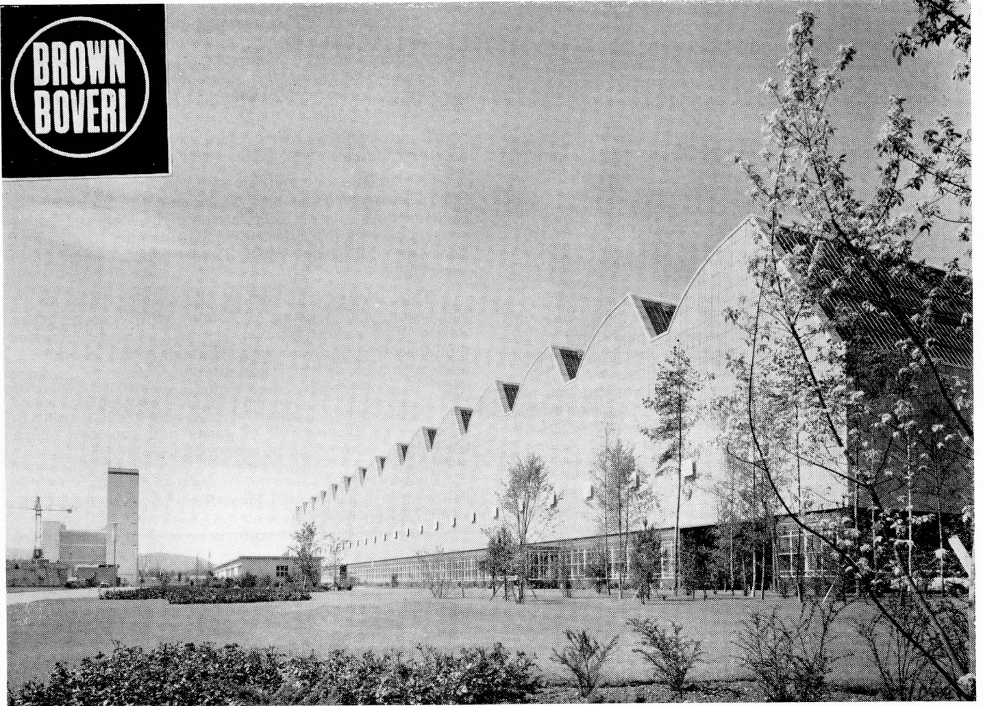
New works at Birr Aargau
