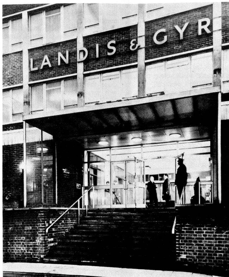
Entrance to Landis & Gyr Administrative Block
