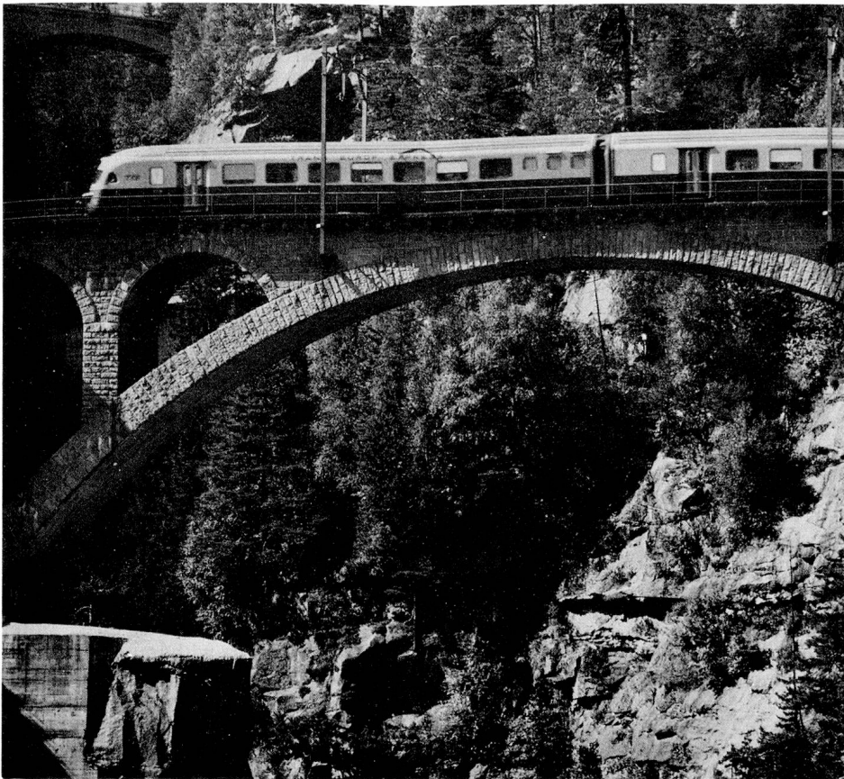
The Gotthard line at Wassen as it climbs over 600 ft. in a huge S-bend, crossing the Meienreuss torrent three times. Here the TEE train "Ticino", on its way from Milan to Zurich, crosses the middle bridge some 230 ft. above the torrent.
