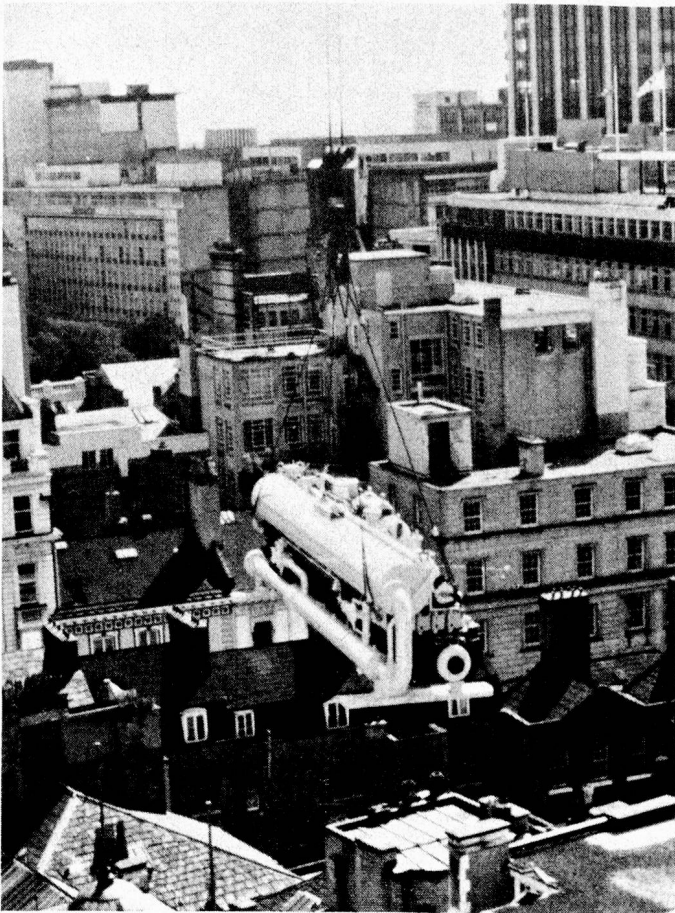
The UNITOP being lowered to the plant room.
