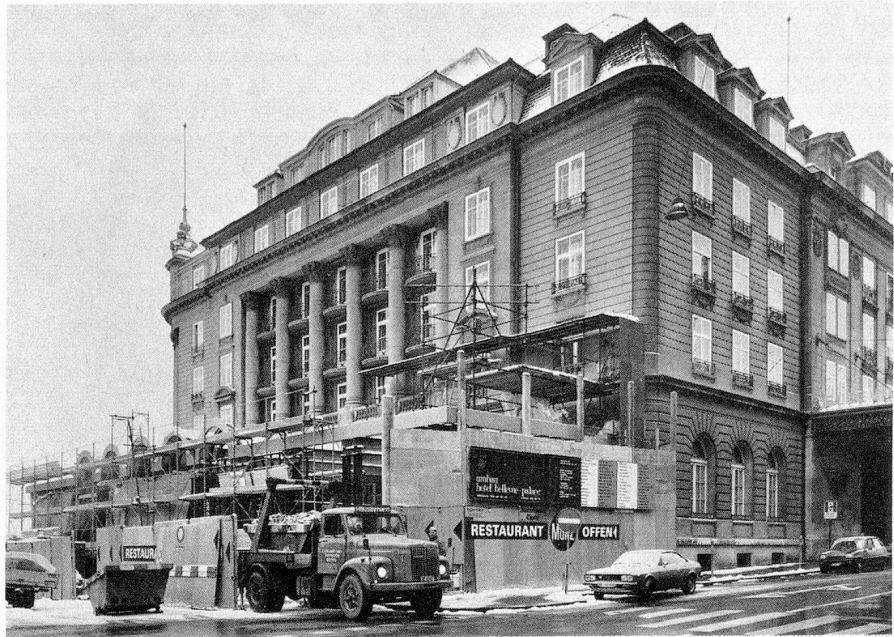
The new "city restaurant" under construction as part of the Sw.Fr. 5.5 million modernisation scheme at Berne's Bellevue Palace Hotel.
