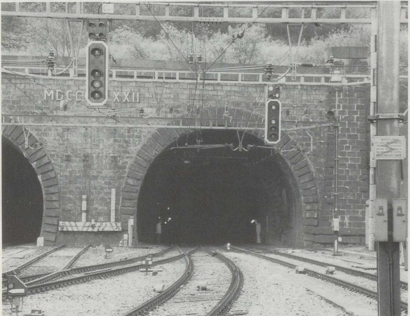
Gantry mounted 4 aspect signals, the Gotthard Tunnel at Göschenen.
