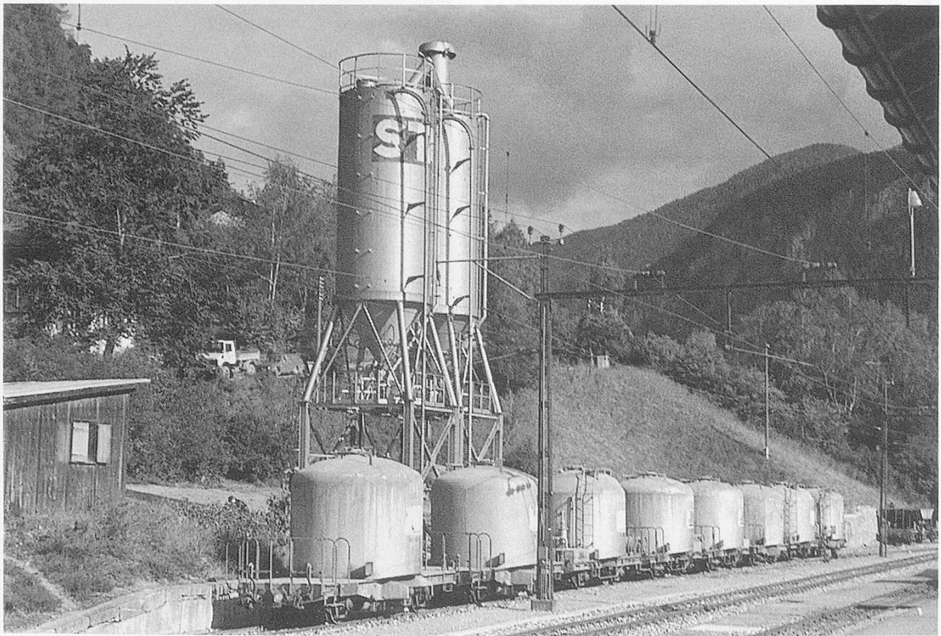
Cement silos with cement train at Tiefencastel, September 1978.
