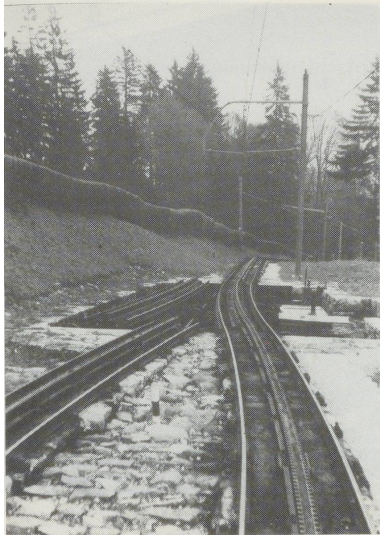
Traverser "points" at Aemsigenalp passing loop.
