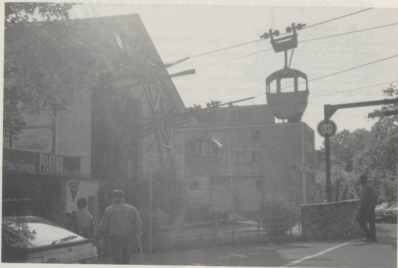
Above : The lower station of the Krienz - Fräkmüntegg gondelbahn : 16 June 1992
