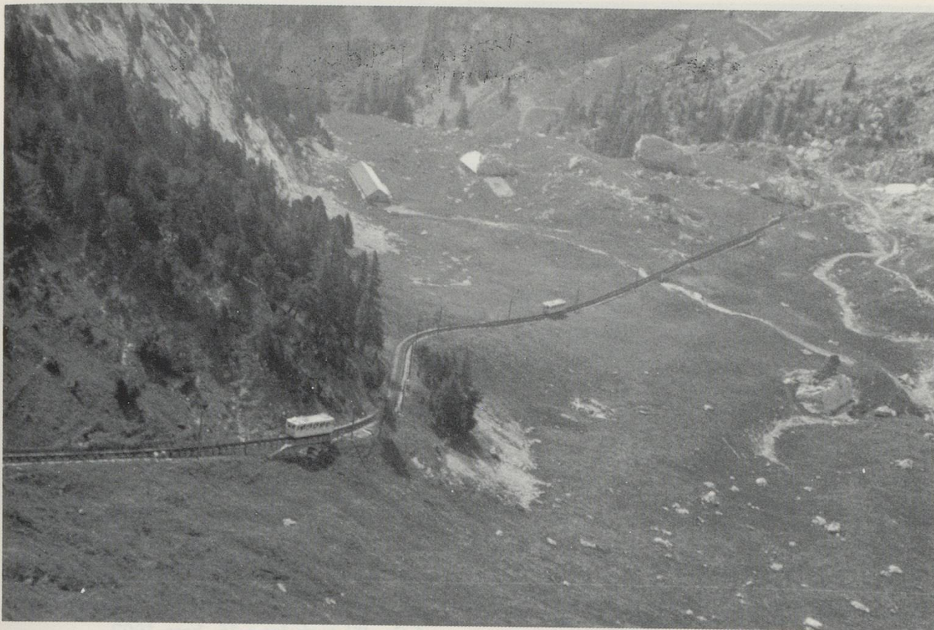
Above : Two railcars in convoy descending the upper section of the Pilatusbahn and crossing the Mattalp, taken from the fourth descending car : 16 June 1992
