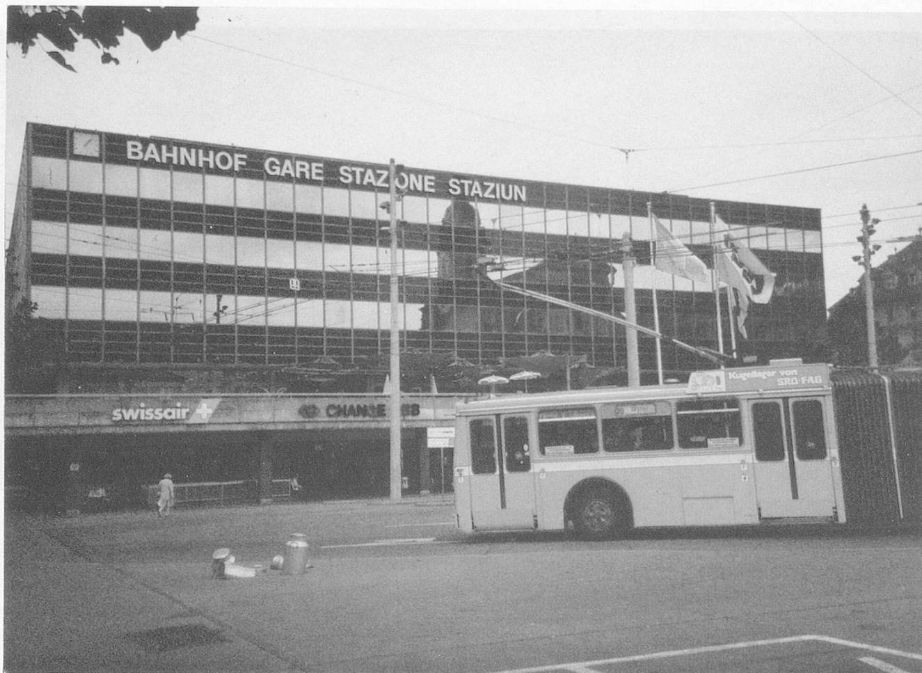
The exterior of Bern station. Note milk churns embedded in the pavement, symbols of Bern's past trade.
