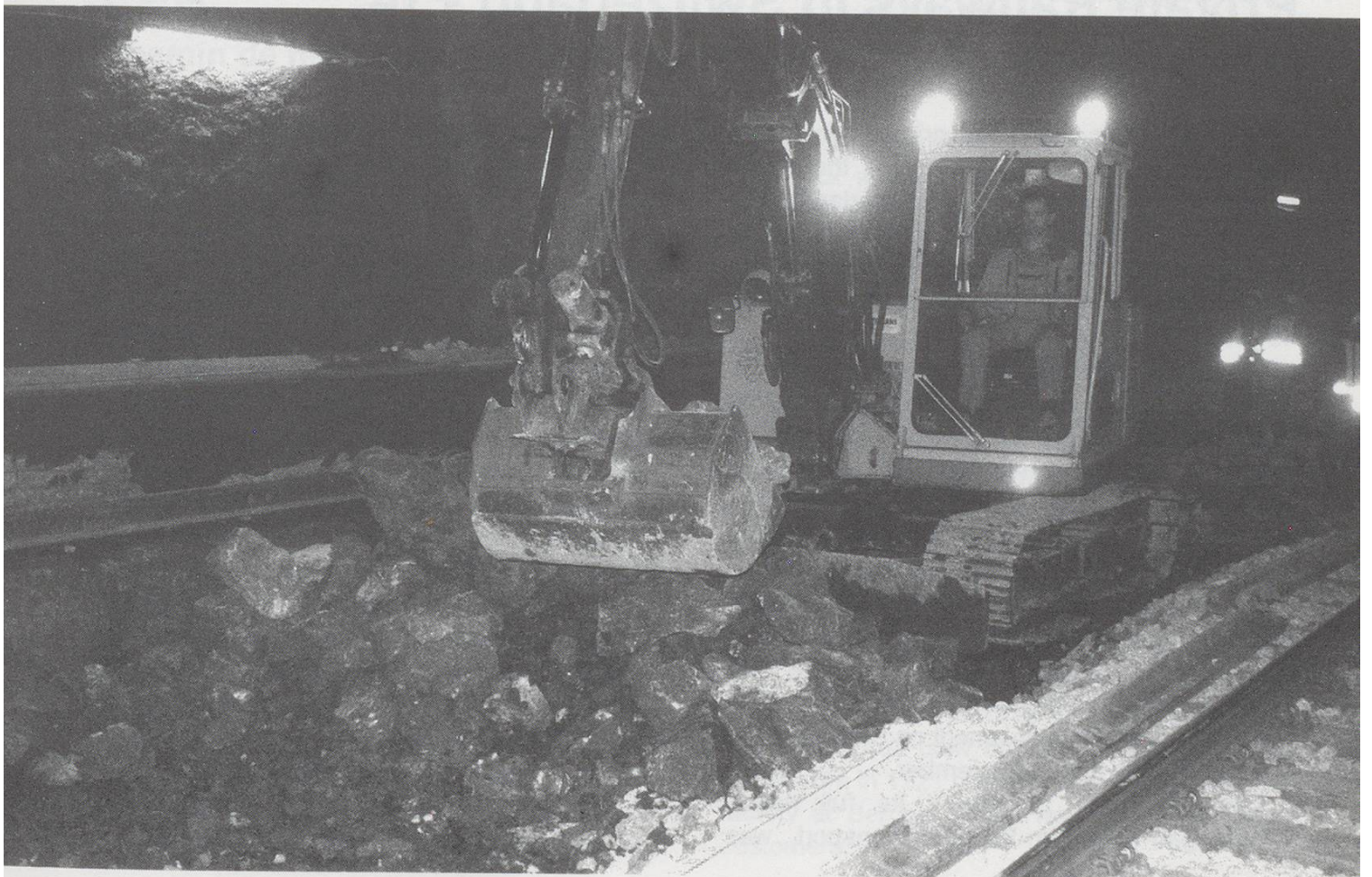
Below: One of loaders at work: look at the close to;erance - the rail on the left is the "running rail".
