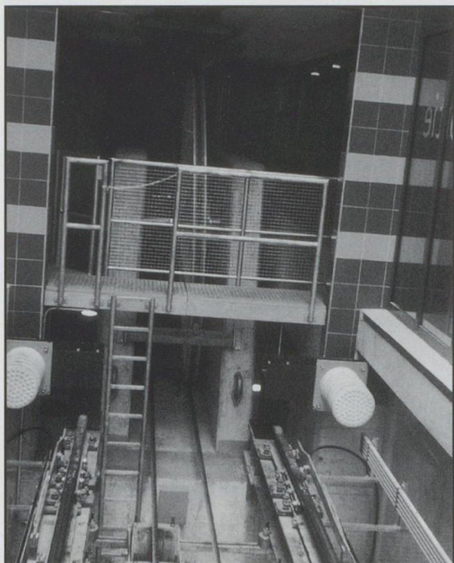
Opening day - lower end - cable wheel, detectors etc.
