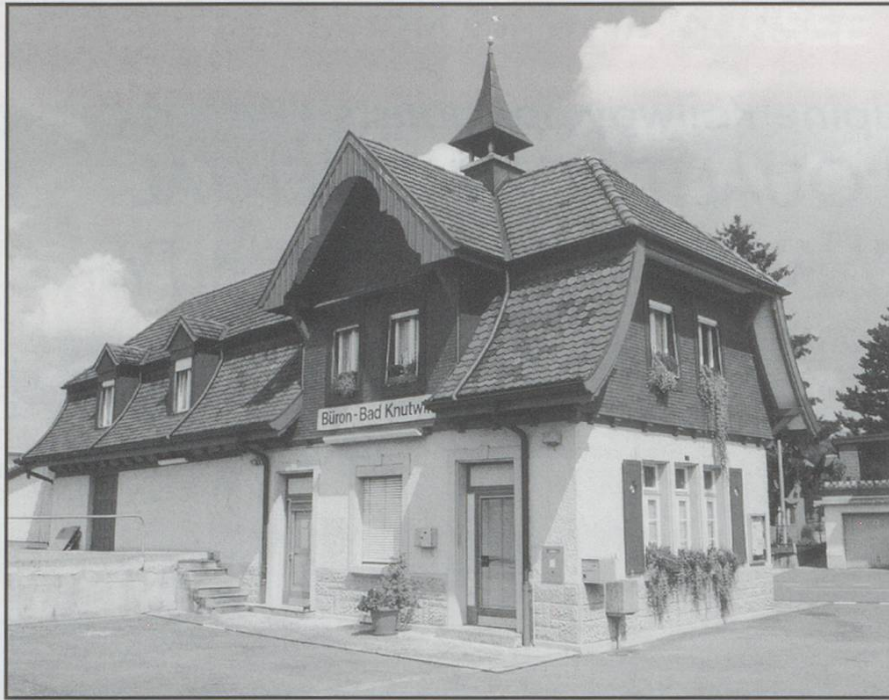
The attractive station at Büron
