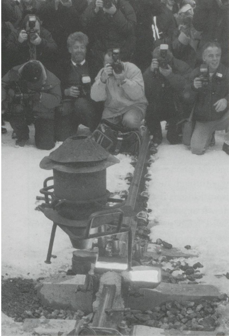
Molten metal flows through to join the rails as the worlds railway press snap in unison. Photo: Chris Harnett
