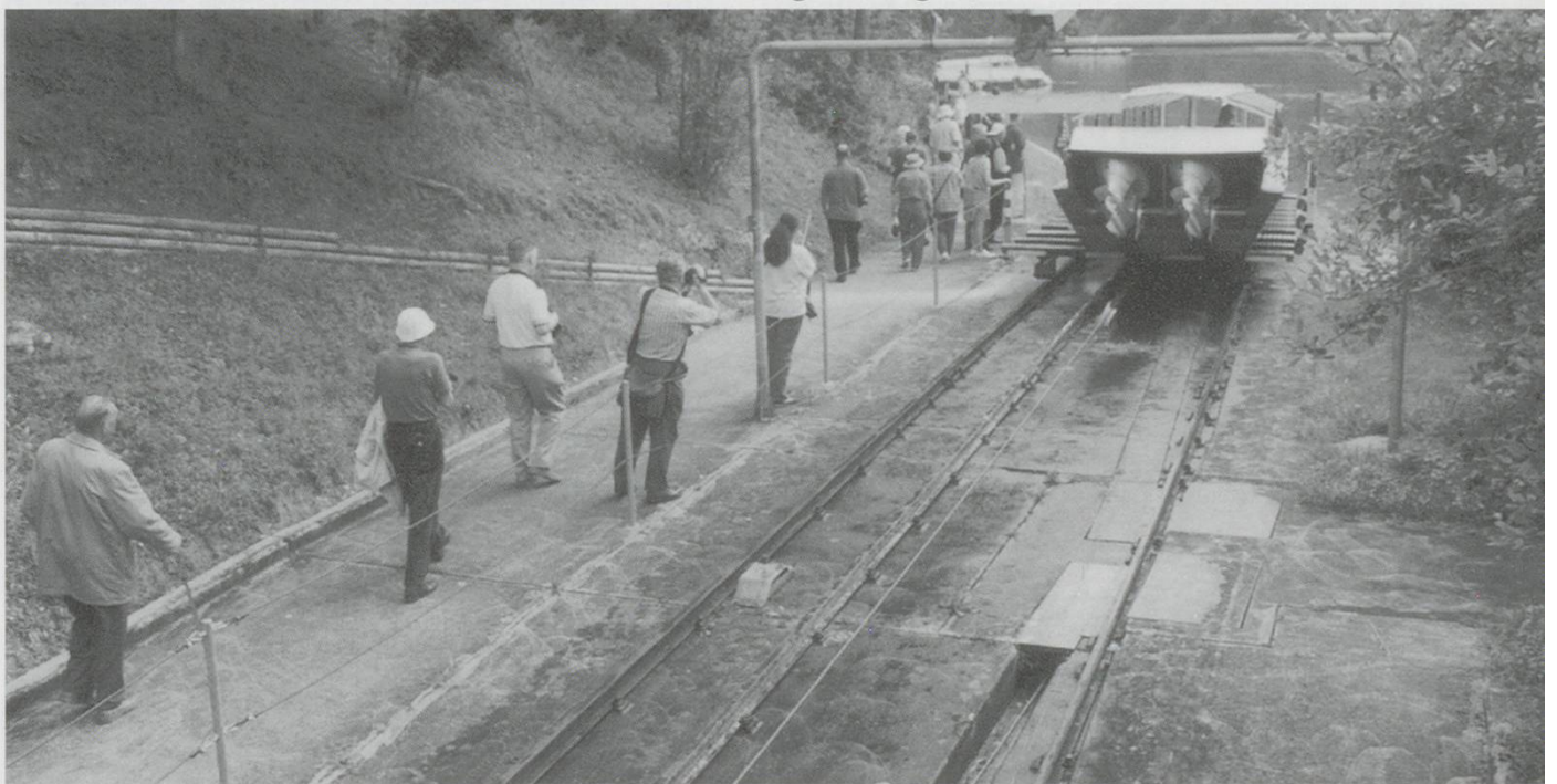
Cradle with boat approaching the water above the weir. Note haulage cable in channels to under track pulleys at lead in to winch (out of sight on right).
