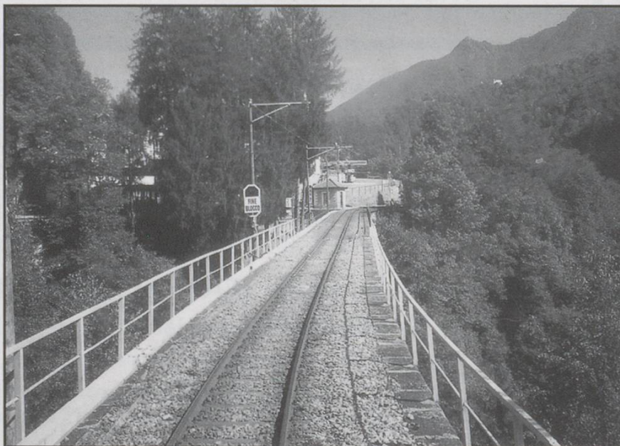
The viaduct at Camedo. 7/9/2000. Photo: Douglas Ellison
