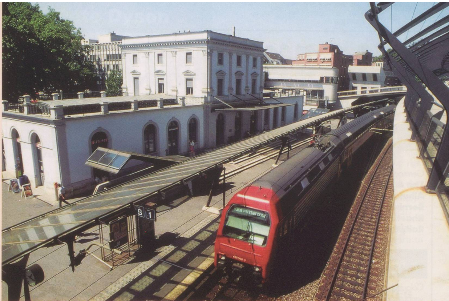
Another view of the old and modern mix at Zürich Stadelhofen. © STS
