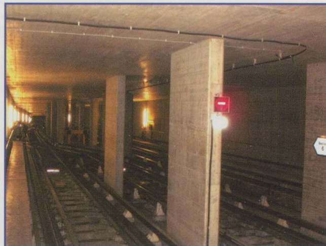
A1:8 incline, and an 80m radius curve, start right at the end of a station. Platform doors are on the left.
