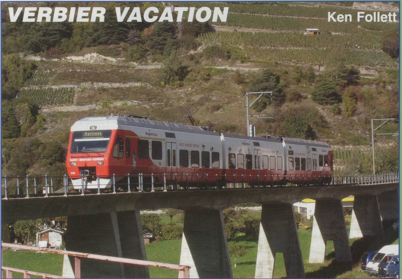
TMR(MO) low floor 'NINA' EMU RABe No.527.513 service from Le Chable on viaduct approaching Sembrancher on 10 October 2006. PHOTOS: Ken Follett.
