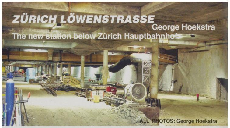
During 2002 – 2004 when the track into the Hauptbahnhof was re-laid, the opportunity was taken to construct part of the new underground station (shown here) in relative ease, before the new track was laid down.
