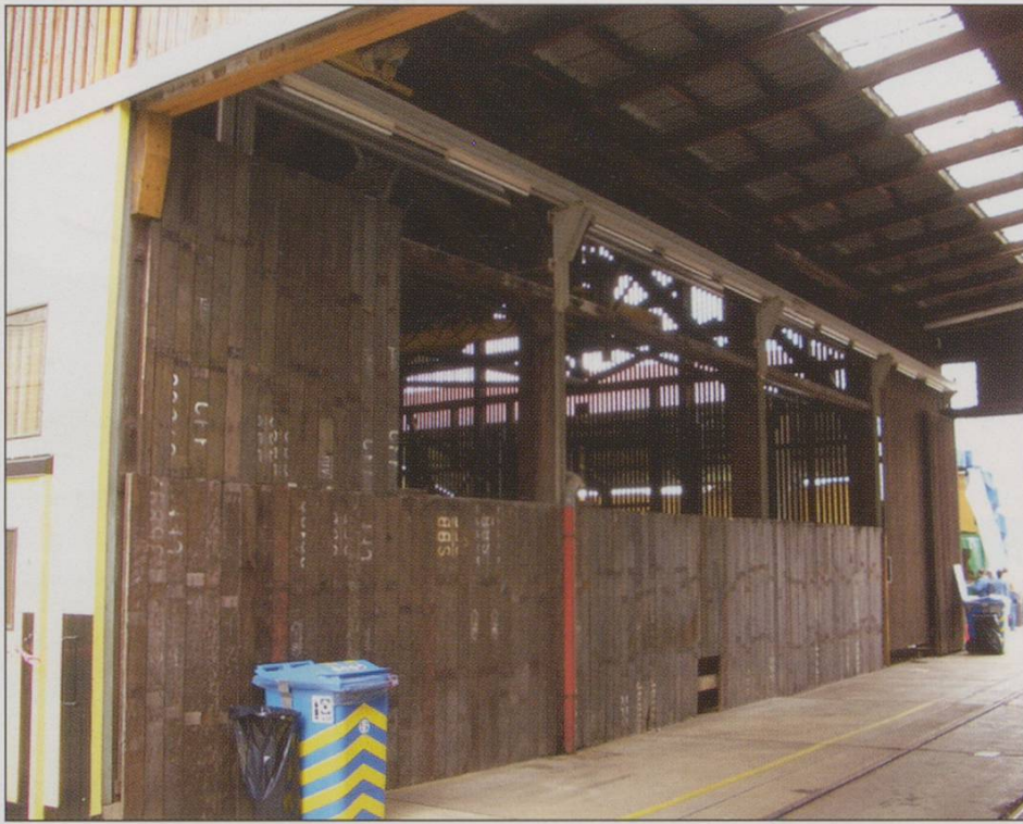
7. Yverdon Works. A windbreak incorporates wooden planks recovered from scrapped wagons, 9/2005.
