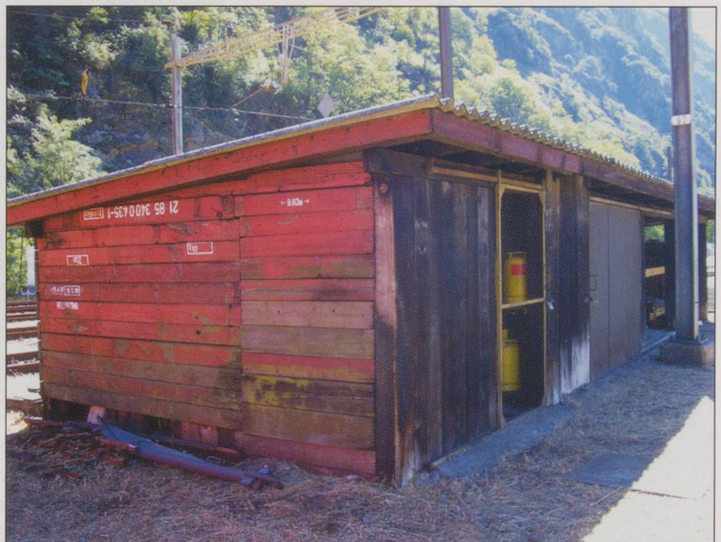
6. Biasca. This small shed was built using material recovered from scrapped wagons, 9/2007.
