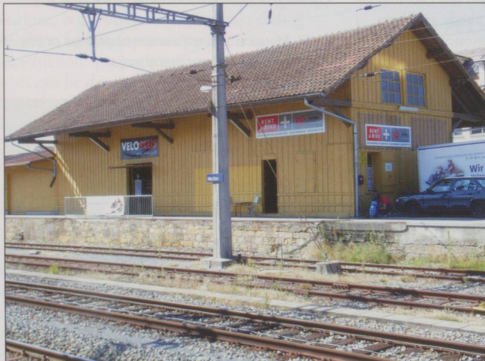
recovered from scrapped freight wagons. This type of ‘internal’ recycling ensures that the railway company largely avoids costs normally associated with the purchase or rent of a new building from the commercial market by keeping the project entirely ‘in-house’. During the ‘Gotthard 150’ event at 5a. Murten. This freight shed now acts as a ‘Velo Station’ for tourists and visitors, 9/2009.
