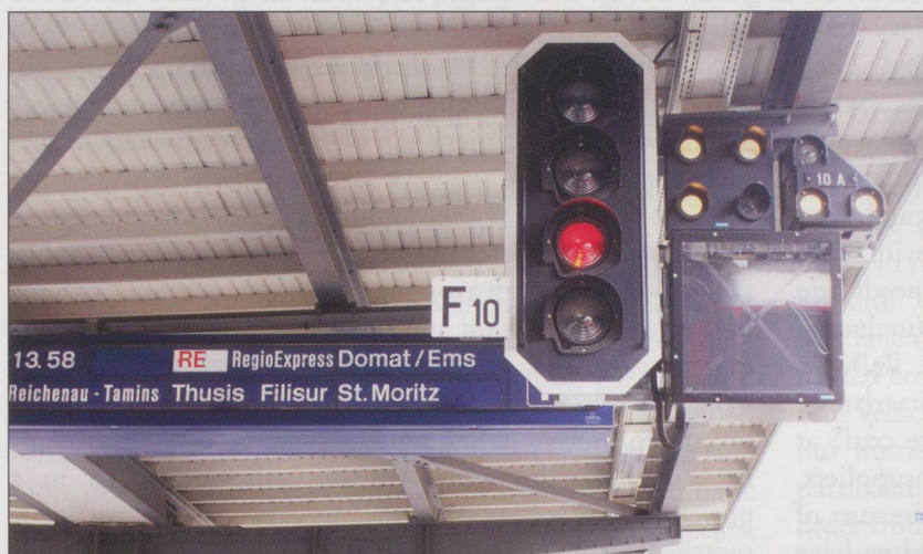
ABOVE RIGHT: A Train Conductor is activating the departure order.
