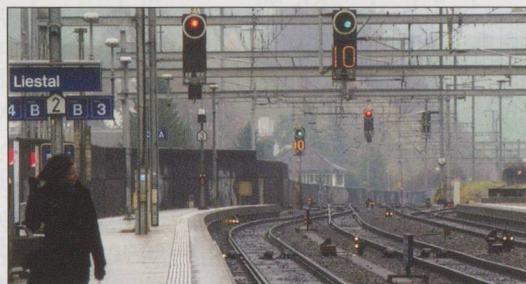
BELOW: Signals at Liestal. Platform 3 signal at stop, the through track clear to enter the section at 100 km. Note also the dwarf signals on the main lines.
