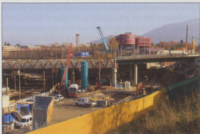
CEVA works at La Praille Yard. Photo: Gordon Wiseman
