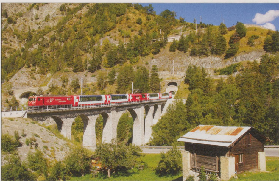
TOP: MGB Deh4/4II No. 93 with east-bound train on Grengiols river bridge - viewed from the hill above the bridge.
