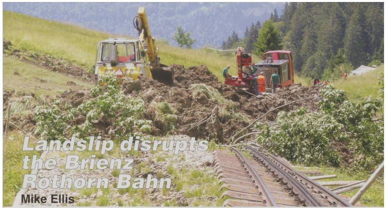
A clear view of just what has happened. The track, is some 3-4m out of alignment, completely free of the trackbed and now buried under a thick layer of clay, trees and boulders.
