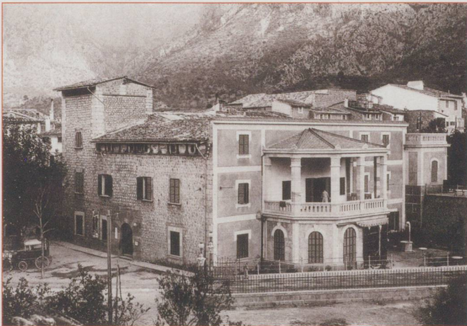
Soller station front. The house as was, but changed to become the station with the booking office, etc. inside.
