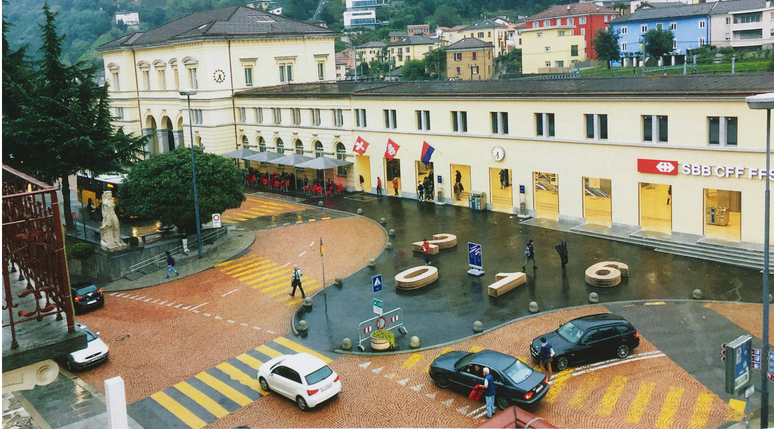
The road side view of Bellinzona station.
