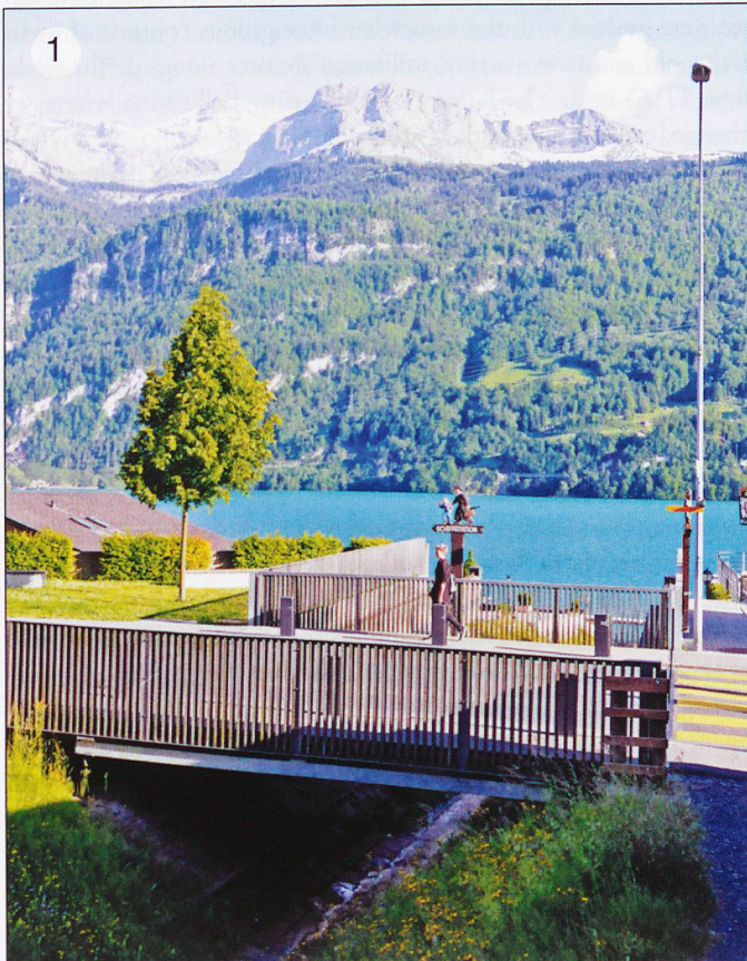
4. This gives a better idea of just how steep the waterway is, and how much extra space for water and debris is achieved by moving the bridge. The controls for the bridge are also in the picture.
