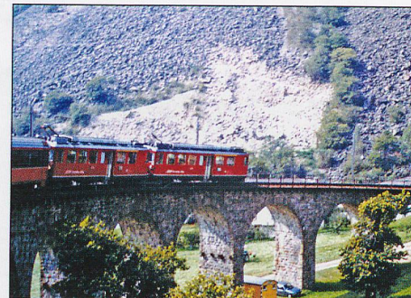
Brusio circular viaduct.
