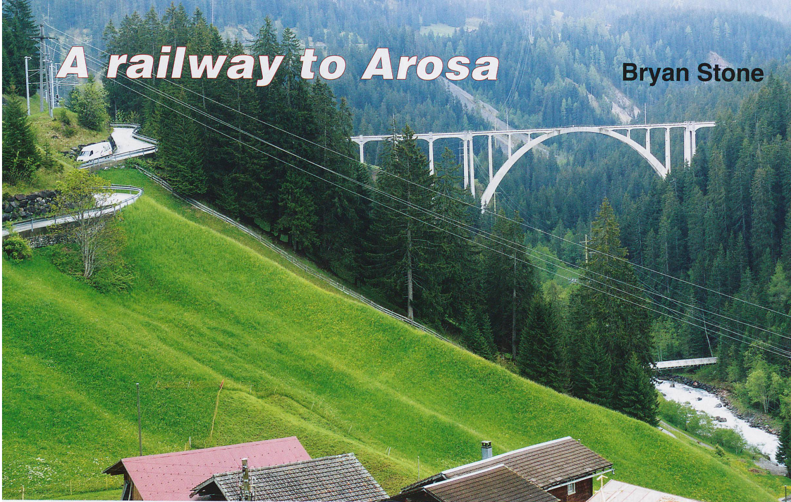
The difficult landscape and the famous Langwies viaduct.
