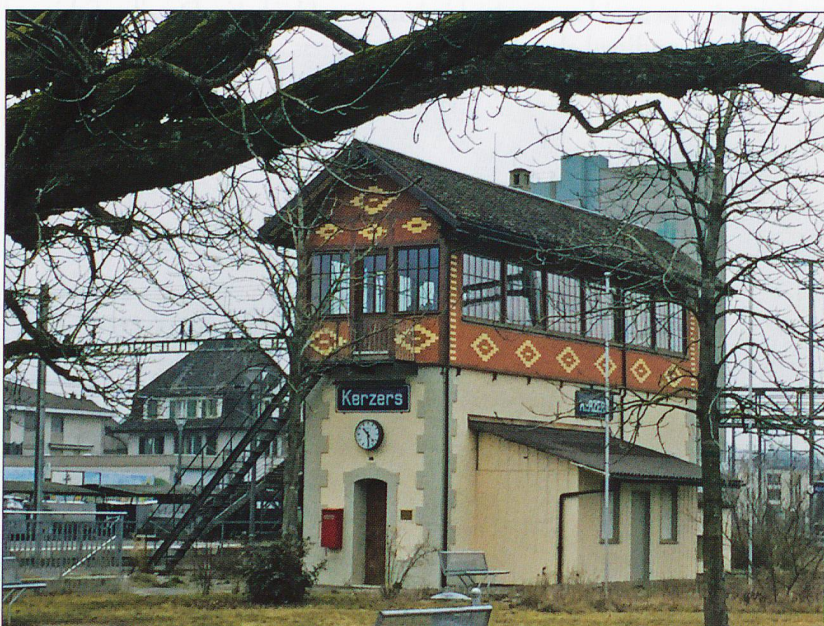
The signal box at Kerzers.
