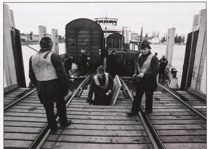
LEFT AND ABOVE: Photographs showing unloading procedures.
