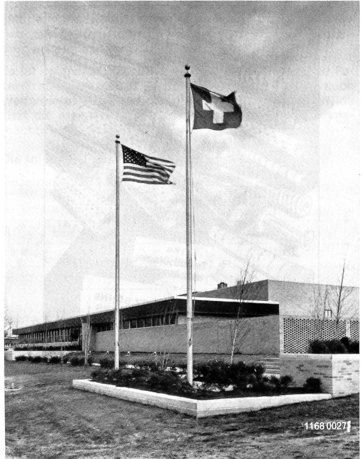
Sulzer-Textile Center in Spartanburg, South Carolina.
