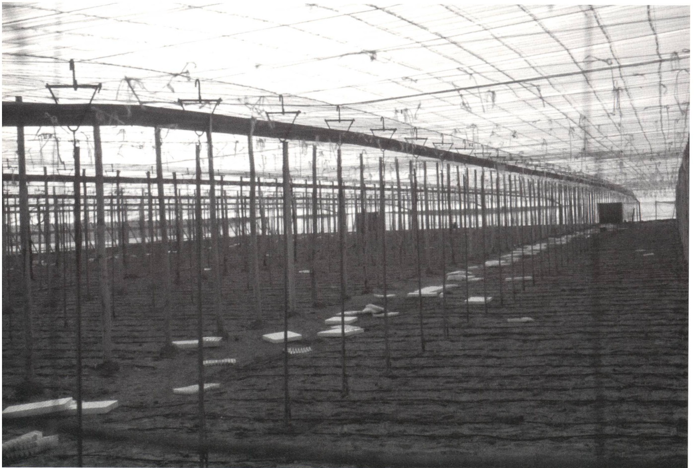
Inside the Membrane
