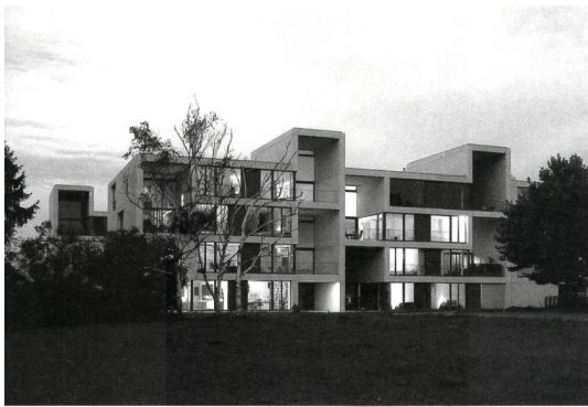
Zapco Ltd., Pile Up am Rhein , Rheinfelden, 2005.
