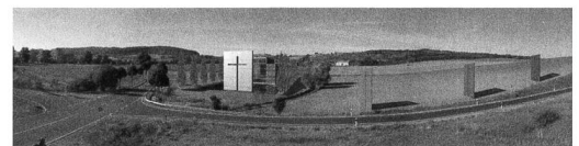
Werkstatt GAW Architects, Containerbasilica , Autobahn A38 Friedland/Rosdorf, Göttingen, 2006.
