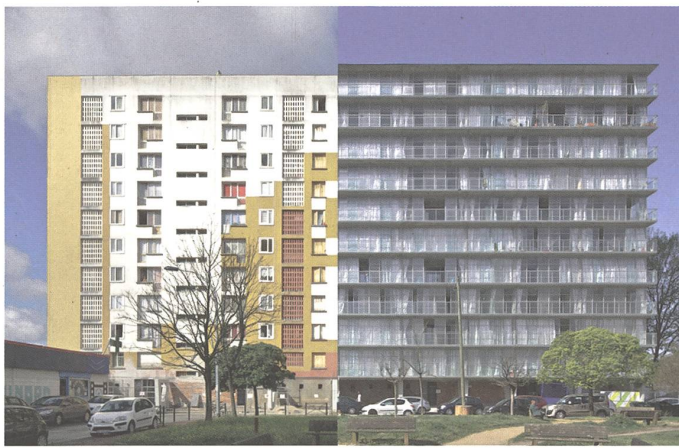
fig. g Transformation of buildings G, H, I, Grand Parc, Bordeaux, France by Lacaton & Vassal, Druot, Hutin, 2016 © Philippe Ruault
