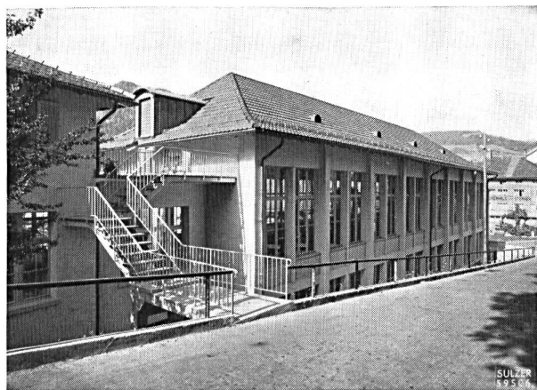
The new premises built in 1950.
