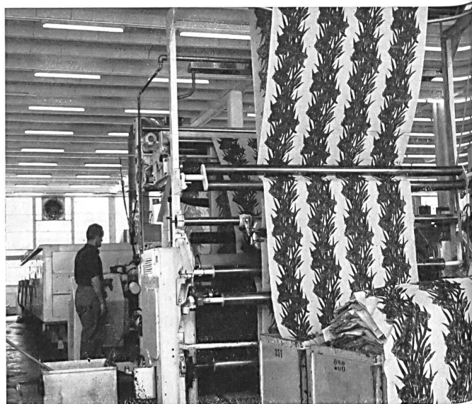
Fabric starting off in a dressing machine
