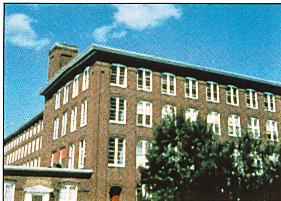
On historic grounds: The Hathaway plant at Waterville/Main.
