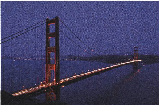
Golden Gate Bridge by night
