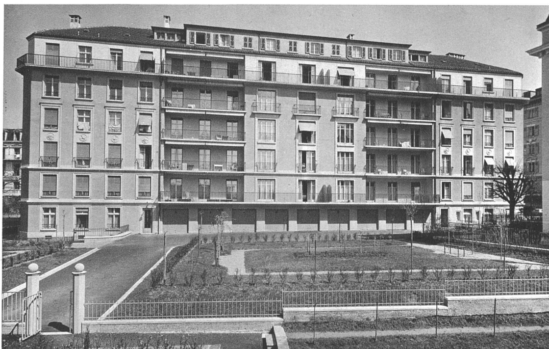
Façade sud, garages
