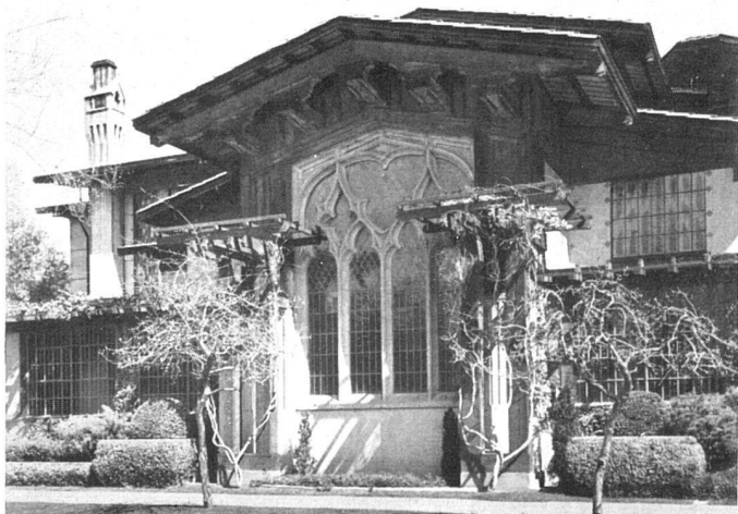
Christian Science Church, Berkeley, Seitenansicht | Façade latérale | Side-elevation
