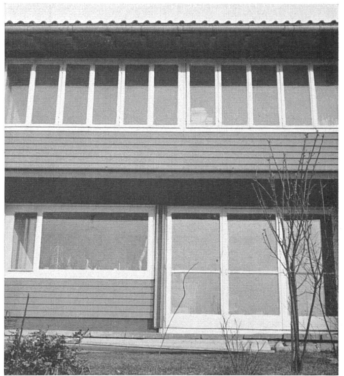
Fassadendetail | Detail de la façade | Elevation detail
