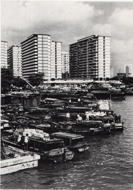
2 Crawford Street Redevelopment am Rochor Canal, Singapore-Ost
