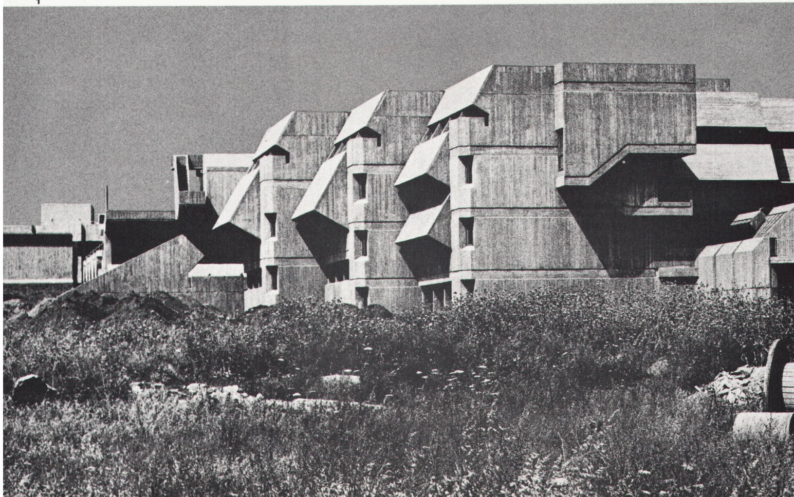
1 General view 2 Bottom view of passageways around the courtyard 3 The inner courtyard 4/5 Workshops
