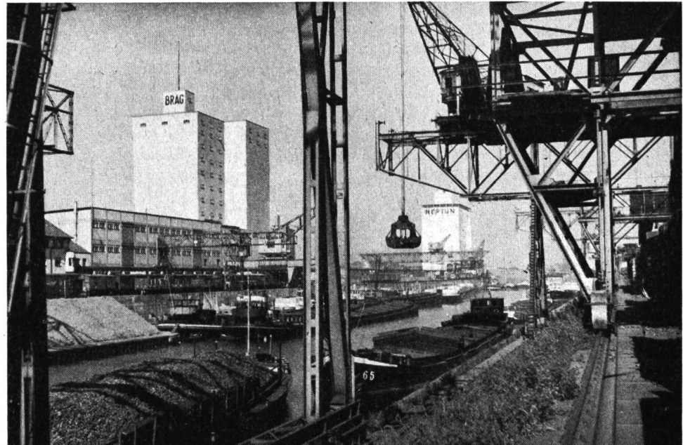
Abb. 6 Hafenbecken II in Basel. (Photo F. Ritter, Basel)
